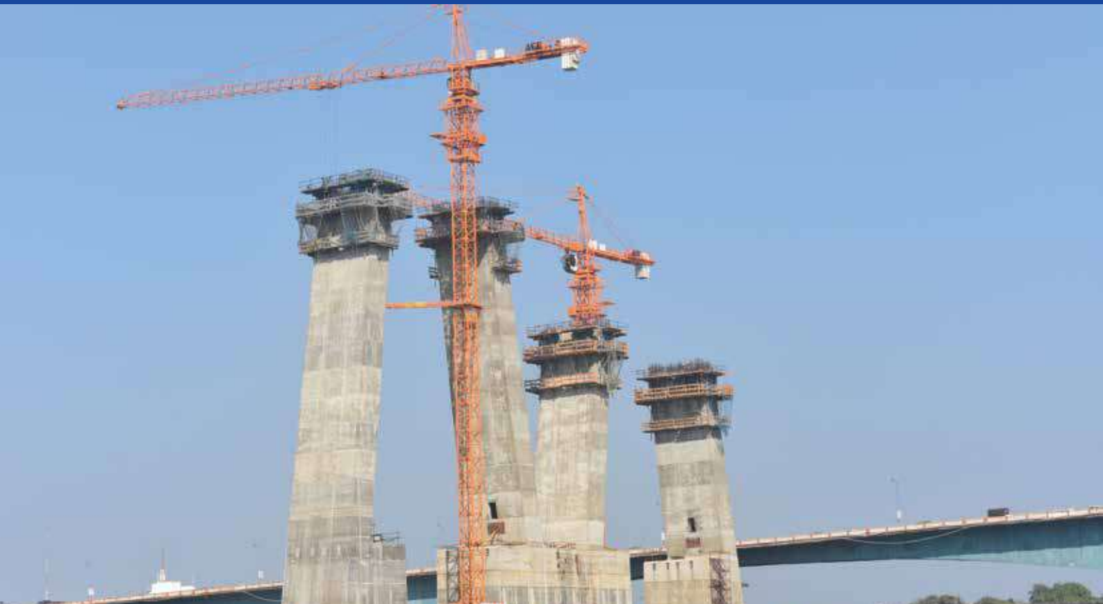
Zuari bridge, Goa
